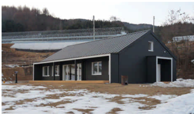
The finished passive house (Photo Yoon-Boum Cho)
